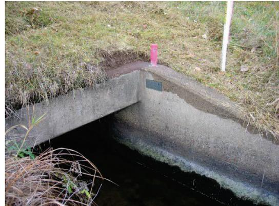
*Figure 5 – WisDOT HMP bronze disk set in bridge abutment*      *Figure 6 – WisDOT HMP bronze disk set in box culvert*
