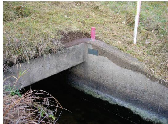
*Figure 6 – WisDOT HMP bronze disk set in box culvert*
