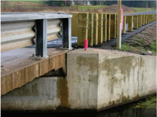
*Figure 5 – WisDOT HMP bronze disk set in bridge abutment*
